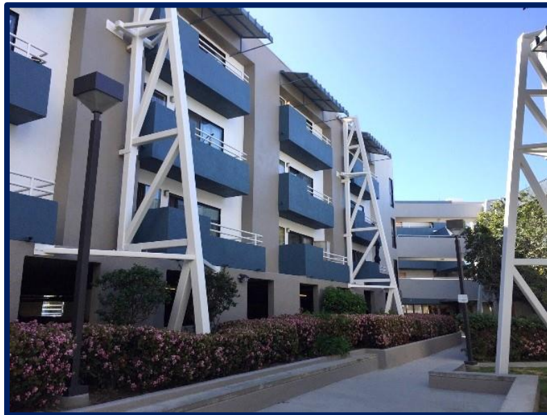
Marina Manor Exterior Improvements
